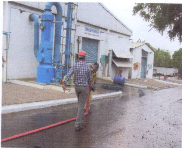
Fixed Mayur water curtain by using SCBA set during emergency
