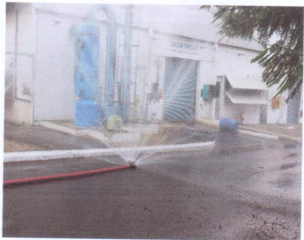
Mayur Water curtain being activated as barrier for UGST area.
